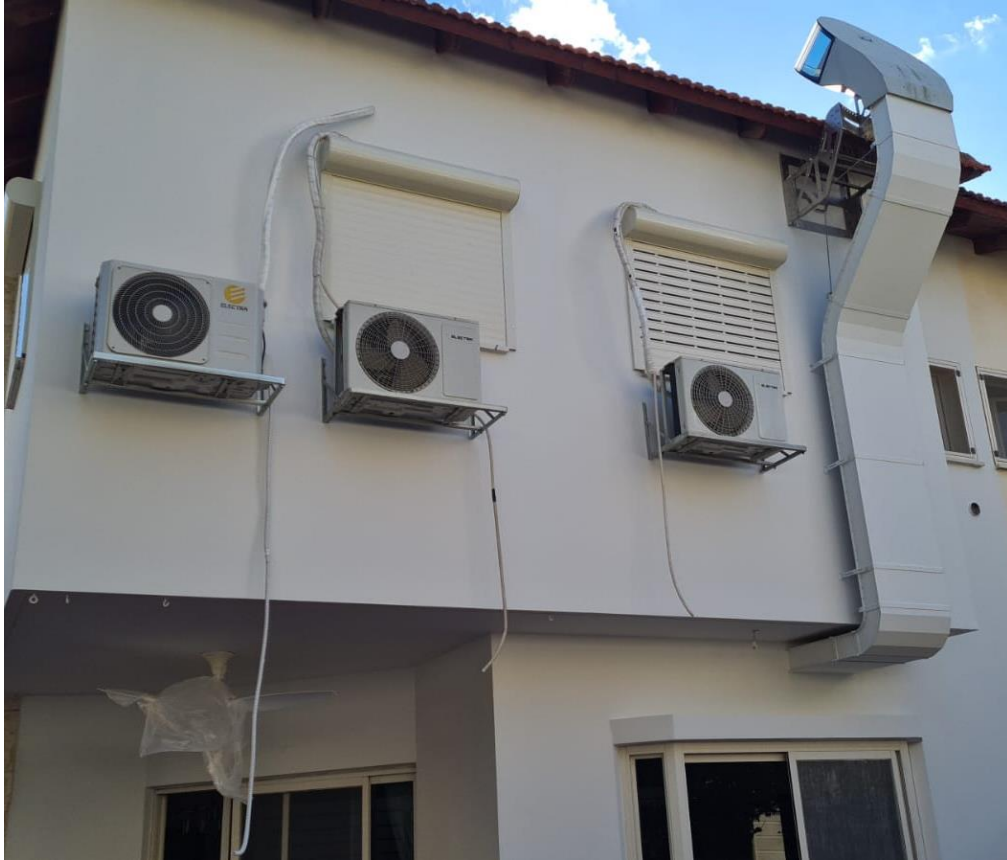
SOLIS fully external Retrofit, no change to the building, North-Side installation.
